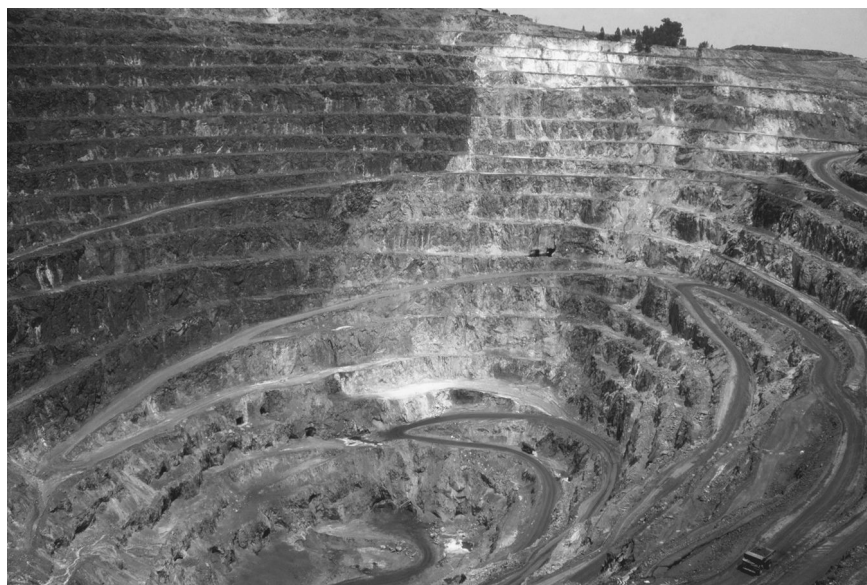
Fig. 1.7. The largest historic copper open-pit mine in Europe: the Corta Atalaya, Rio Tinto, Huelva, Spain
