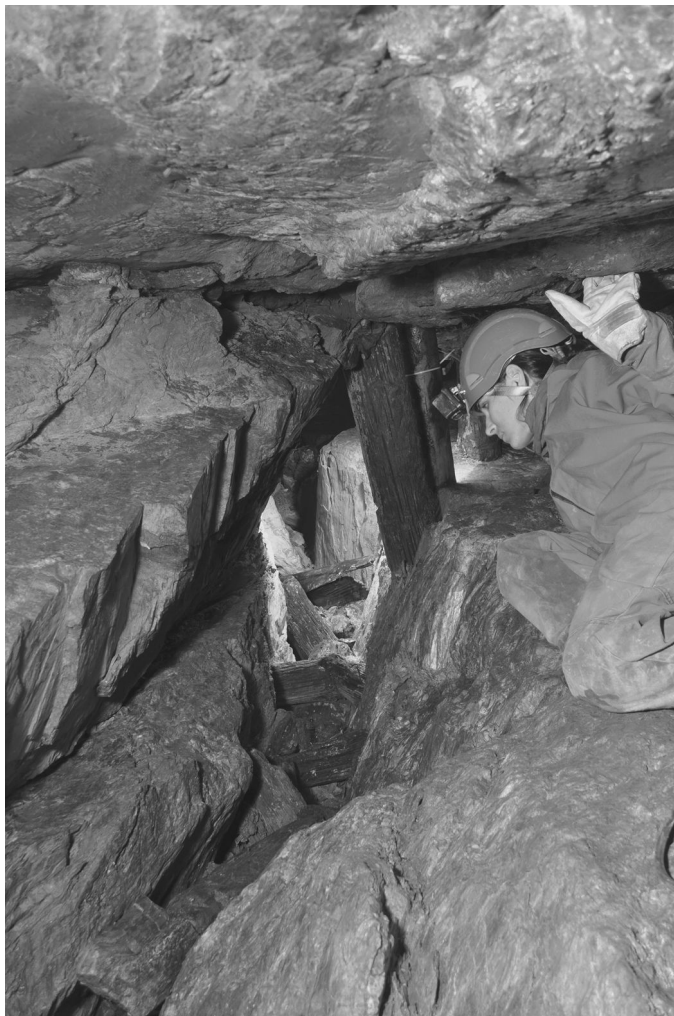
Fig. 7.7. Wood stemples from Bronze workings exposed in the Arthurstollen gallery, Mitterberg
