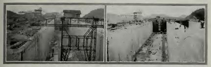
Miraflores Locks. Concrete-mixing plant in the distance. The specks at the bottom of the lock in right-hand view are men.
