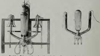
Rectifier Tubes, with and without holder-Sacramento Substation.
