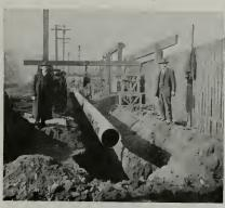
1000 pounds of pipe hang on a welded joint.
