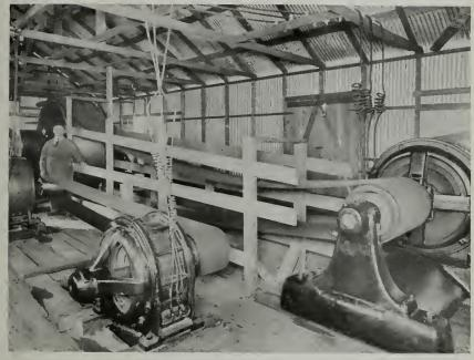
Power-house, showing 12-foot compressor belt-driven to 200 h.p. motor, also motor-driven generator.
