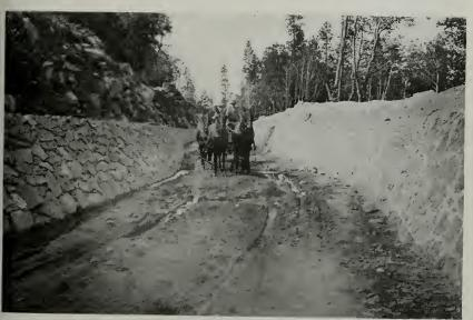
Upper end of Drum canal, fourleen and one-half feet wide, with masonry lining.
