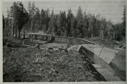
Flume near Drum forebay, showing concrete inlets and outlets.
