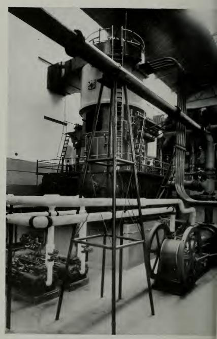
The new 15,000 K. W. turbo-generator installed at station "A," San Francisco.
