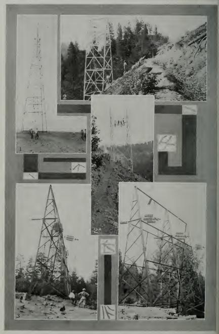
Various types of towers. Fig. 1 shows method used in building up high towers; Figs. 2 and 2a are of snow towers on steep hillsides; Figs. 3 and 4 depict special towers on long spans, Greenhorn Creek and Steep Hollow. In Fig. 3 Mr. Downing is seated by the tower, with Mr. Steele standing beside him.
