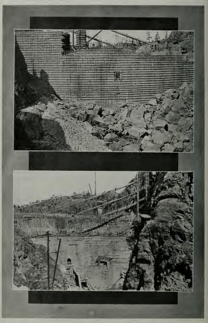
Views of Spaulding Dam in course of construction. That at the top is the upstream face of the dam, showing the unstripped concrete forms. The lower picture shows the downstream face of the dam, with three lines of concrete-distributing chutes. The opening on the left is the inspection tunnel to the drains, weepers, etc. The dam as shown here is 150 feet above bedrock.
