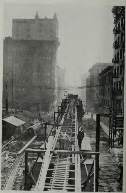
Constructing the Stockton street tunnel. Looking back toward the approach at Sutter street. Picture shows the dump cars running on incline tracks to the bunkers.
