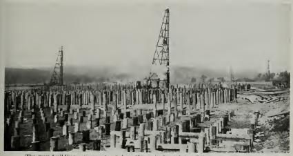
The way buildings are constructed on the waterfront lots. Piles being driven for the foundation of the Transportation Building.
