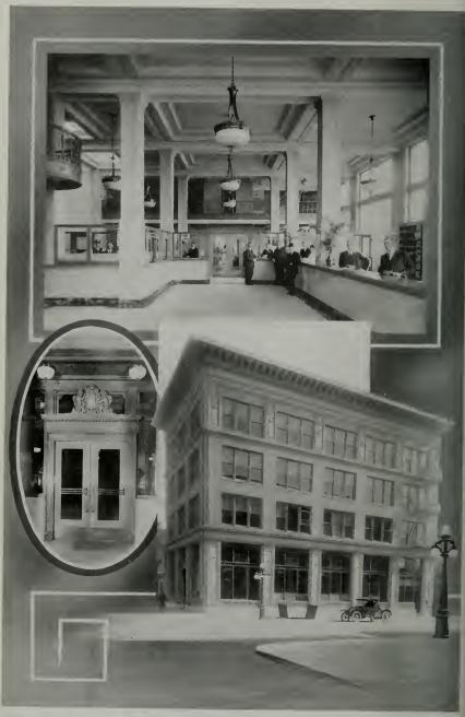
The new "Pacific Service" building in Sacramento. It is situated at Eleventh and K streets and represents the most modern type of office building, four stories high and constructed of reinforced concrete, faced with brick and terra cotta. The architectural design is Italian Renaissance, adapted to modern requirements. Note the ornamental entrance and the spacious public offices on the ground floor.
