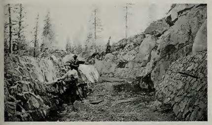
Masonry lining of a portion of Drum Canal. This section passes through huge boulders of granite.
