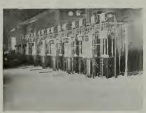
Eight complete 100-light Mercury Arc sets, Sacramento Substation. For cooling purposes the tubes are immersed in oil in small tanks at rear of panel board.
