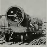
Discharge controlling valves for use at Spaulding dam.
