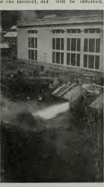
Water discharge from Drum power-house checked by tail-race baffles.
