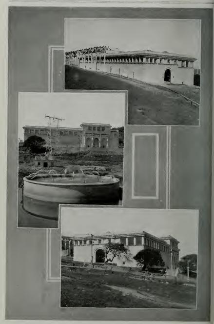
Upper picture gives a rear view of Cordelia substation from the south end, showing the system of pole switches; the center is a front view of the substation, with cooling pond and pump-house in the foreground; the lower shows south end and entrance of the building.
