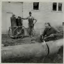
Welding by the oxy-acetylene process.
