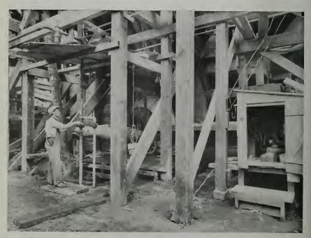
Motor-driven concrete mixer used in constructing the tunnel. "Pacific Service" drives the motor.
