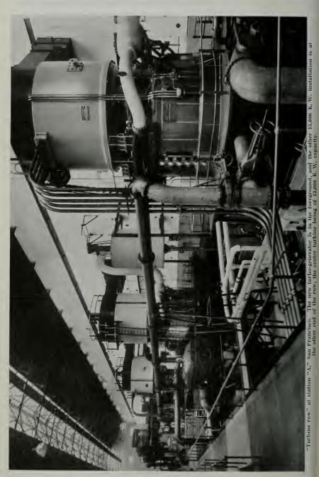
bine are the seven stages, and the extremely large condenser shell. Our other vertical turbines have but five stages, with the single exception of the installation of 1912, which has six, and while the new turbine has exceeded the others in the number of stages, this has been accomplished without any material increase in height.
