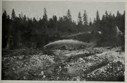
Washing gravel-bank with a monitor to procure gravel for tower foundations.
