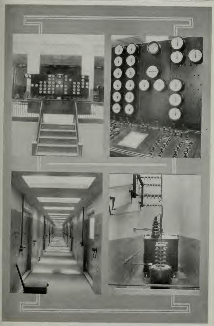
Views of the interior of Cordelia substation. The upper left picture shows the main control-board; the upper right gives a detail view of the same. The view at lower left is of the passage between rows of 60,000-volt oil-switch cells, that at lower right is of an 100,000-volt oil-switch, with current coil.
