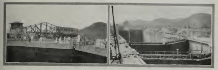
Miraflores Locks. Left—Emergency dam. Right—Protective gate; in foreground, main and intermediate gates; control tower in distance.
