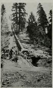
Looking along Drum Penstock No. 1, from an anchor above the power-house. Showing the 54 in. pipe on a slope of 40 degrees.
