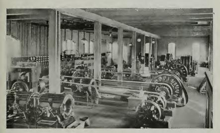
Interior of Sacramento substation. Arc machines, motors and countershafting in foreground, previous to removal.
